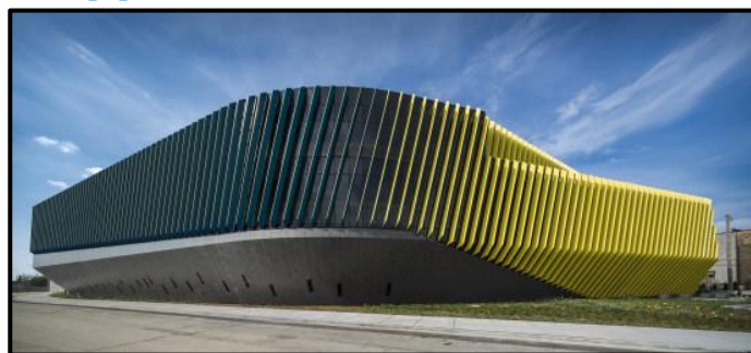
THE APPARENT COLOR OF EL CENTRO CHANGES FROM YELLOW TO BLUE AS ONE DRIVES PAST DUE TO ITS DENSE FIN FACADE. (COURTESY JGMA/LISC)
